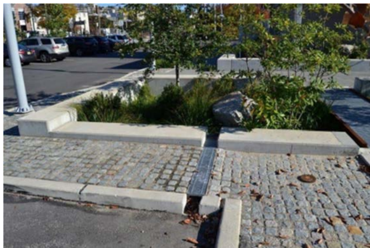
Figure 3: Represents the Planter is designed to Receive and filter Stormwater Runoff from the parking lot.
